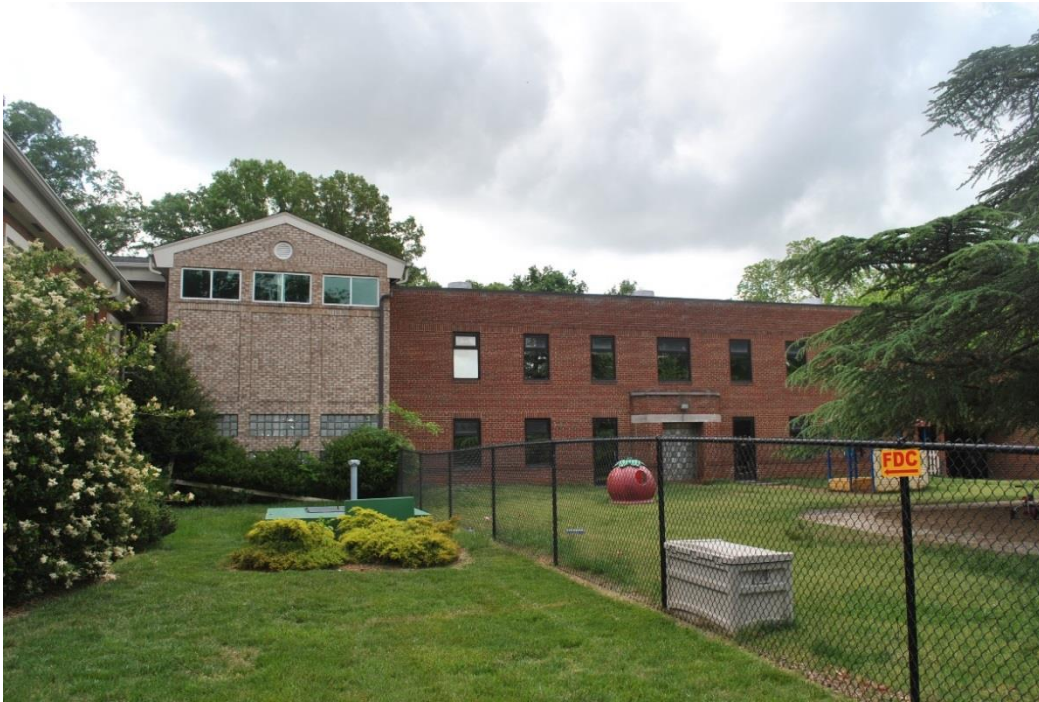
Former Matthews United Methodist Church (116 Ames Street), Rear Educational Buildings, Looking Southeast From North Ames Street.
