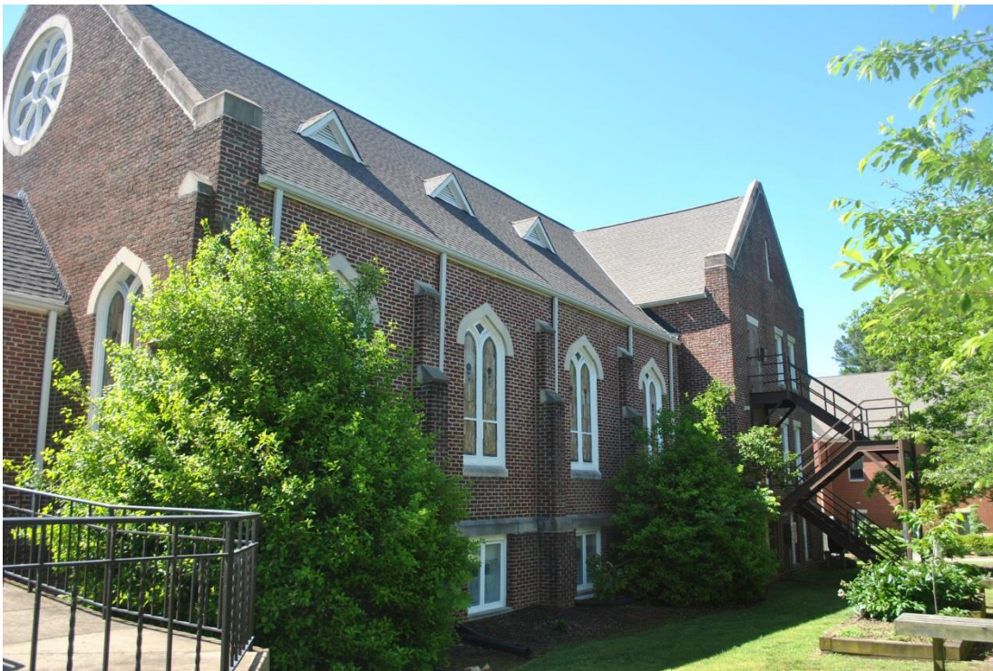
Matthews Presbyterian Church, Side (West) Elevation, Looking South.
