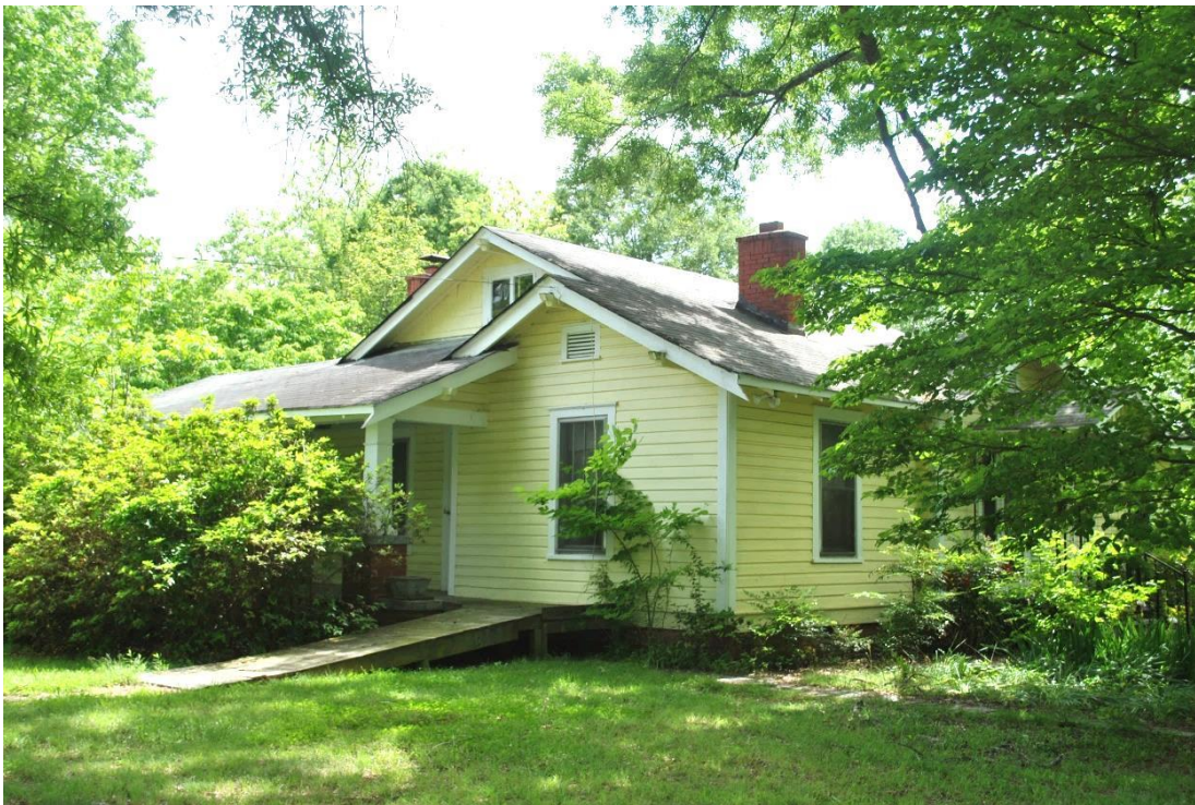
House, 132 South Ames Street, Matthews, Looking East.
