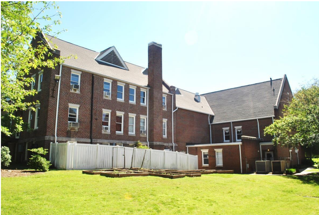
Matthews Presbyterian Church, Rear Classroom Wing, Rear (South) Elevation, and 1976 Classroom Building (Right), Looking Northeast.
