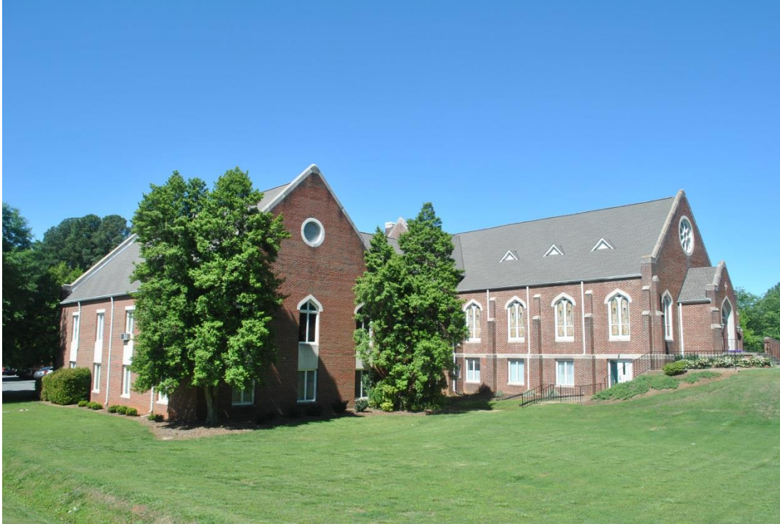
Matthews Presbyterian Church, Side (East) Elevation and 1976 Classroom Addition, Looking Southwest.
