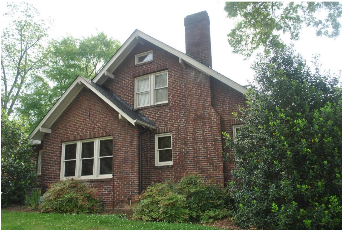
Orr House, Side (West) Elevation, Looking East.
