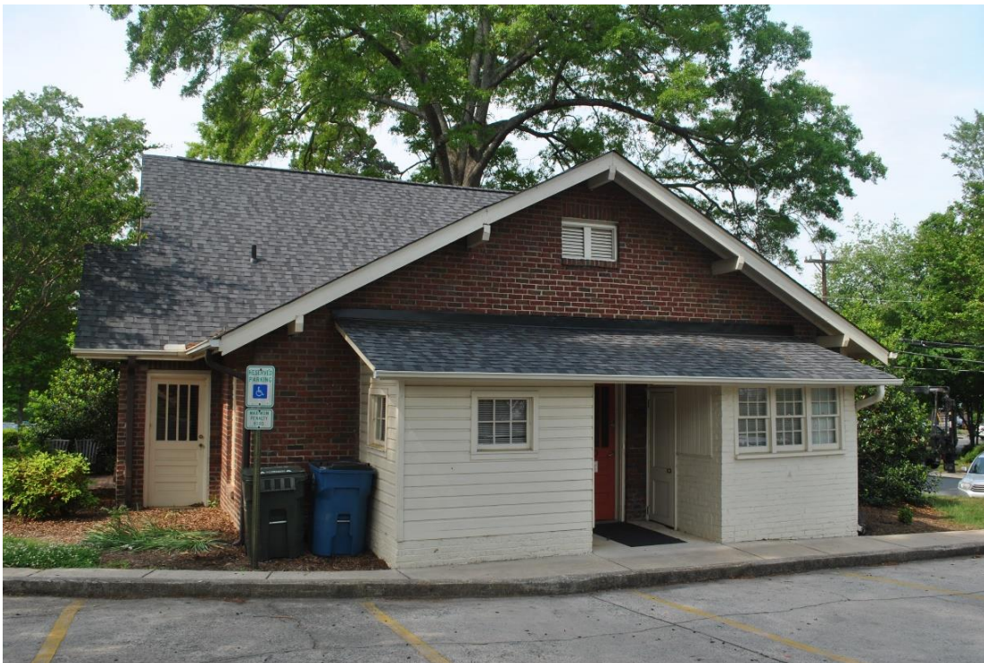
Orr House, Rear (North) Elevation, Looking South.
