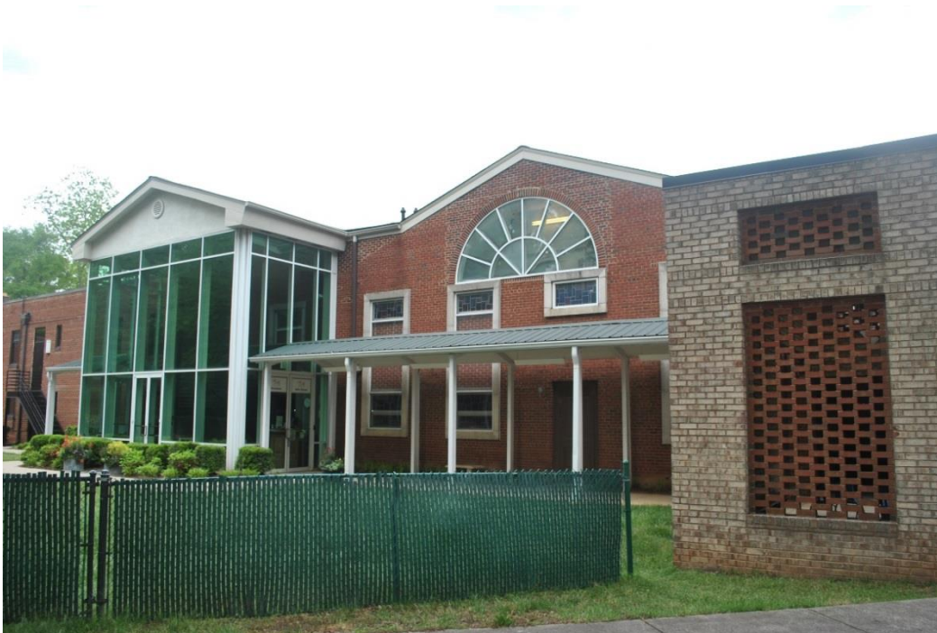
Former Matthews United Methodist Church (116 Ames Street), Rear (East) Elevation, Looking West.
